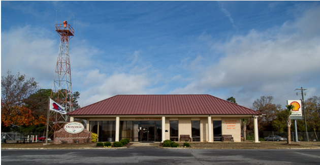
Orangeburg Municipal Airport Terminal
